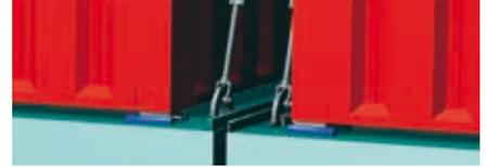
*Dovetail foundation in channel*
