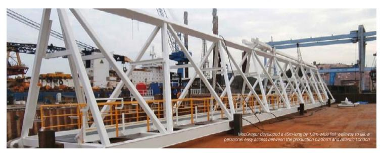
MacGregor has provided the vital connection that allows personnel to move safely between a production rig and a temporary accommodation platform
