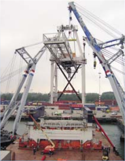
The pontoon is being manoeuvred underneath the crane. The bogies on rails on deck of the pontoon. The new blue portal beams that span 20m.
