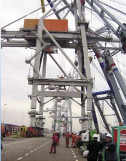
Lifting the crane. The 'splitting-point' of the legs is the lower part of the extension pieces.
