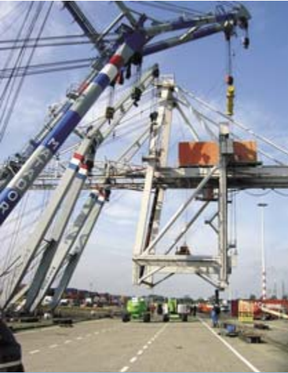
Here, the original extension pieces are removed from the crane.
