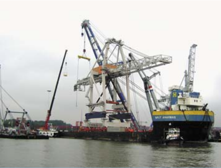
The result: a crane of the same height, but with a railspan of 20m instead of 15m.
