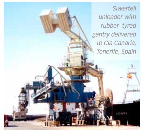
Siwertell stationary unloader operating in the heart of Westhafen, Germany
