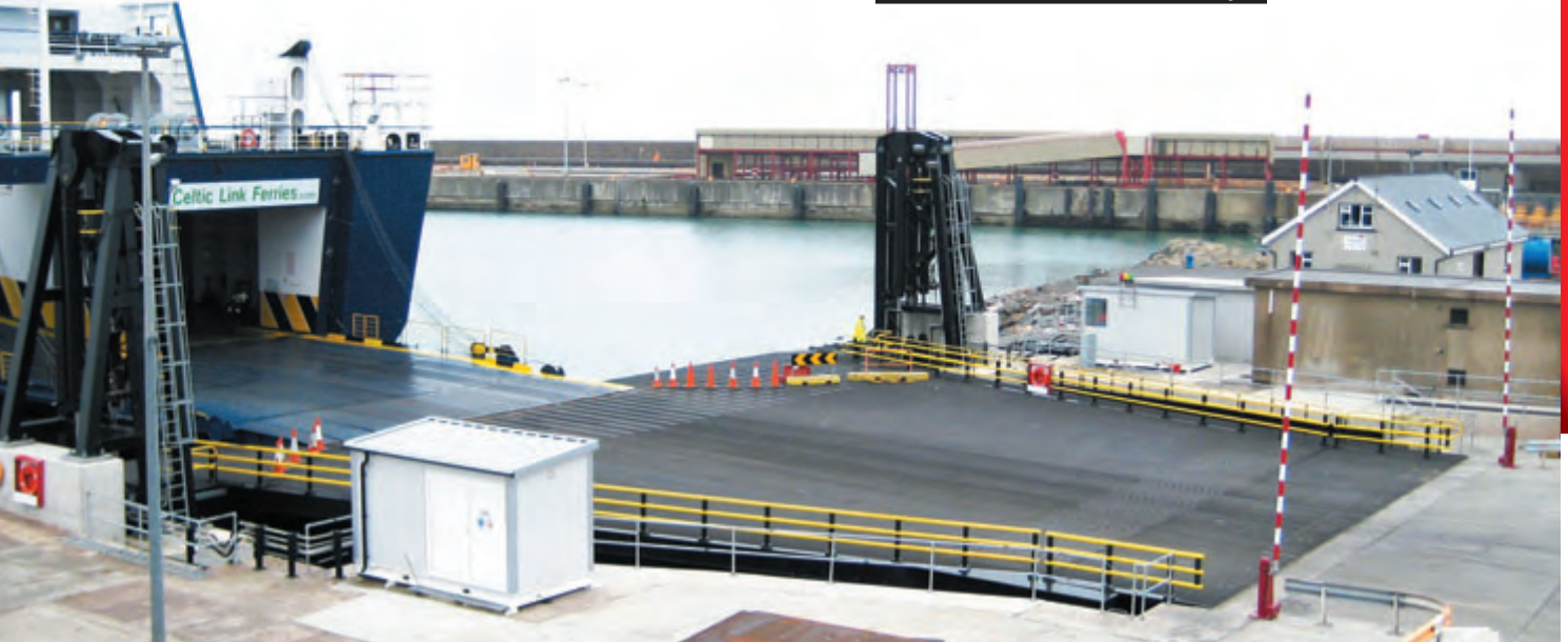
THE 30M-LONG LINKSPAN for the Rosslare ferry port is big for an articulated ramp: its ramp interface is 34m wide at the seaward end and 20m wide at the shoreside end
