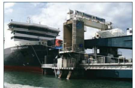
Shore linkspan extended by two outer ramps for two-tier access to feed traffic flows directly to two deck levels.
