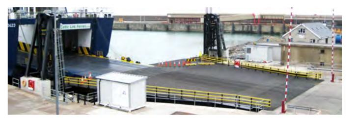
The linkspan is large for an articulated ramp. The seaward ramp interface is 34m wide and the ramp is 20m wide at the shoreside end. It is 30m long in order to cater for the local tidal conditions as well as most ships' thresholds.
